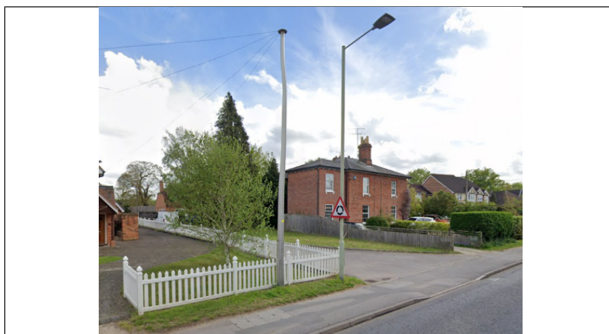
Electricity Pole & Lamp post (Google Street View)
